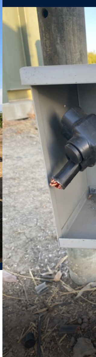
A COP-R-LOCK device is installed on a rural irrigation pump to deter copper wire theft. The tamper-triggered system sends real-time alerts and activates alarms, giving law enforcement a critical window to respond before thieves can flee.
